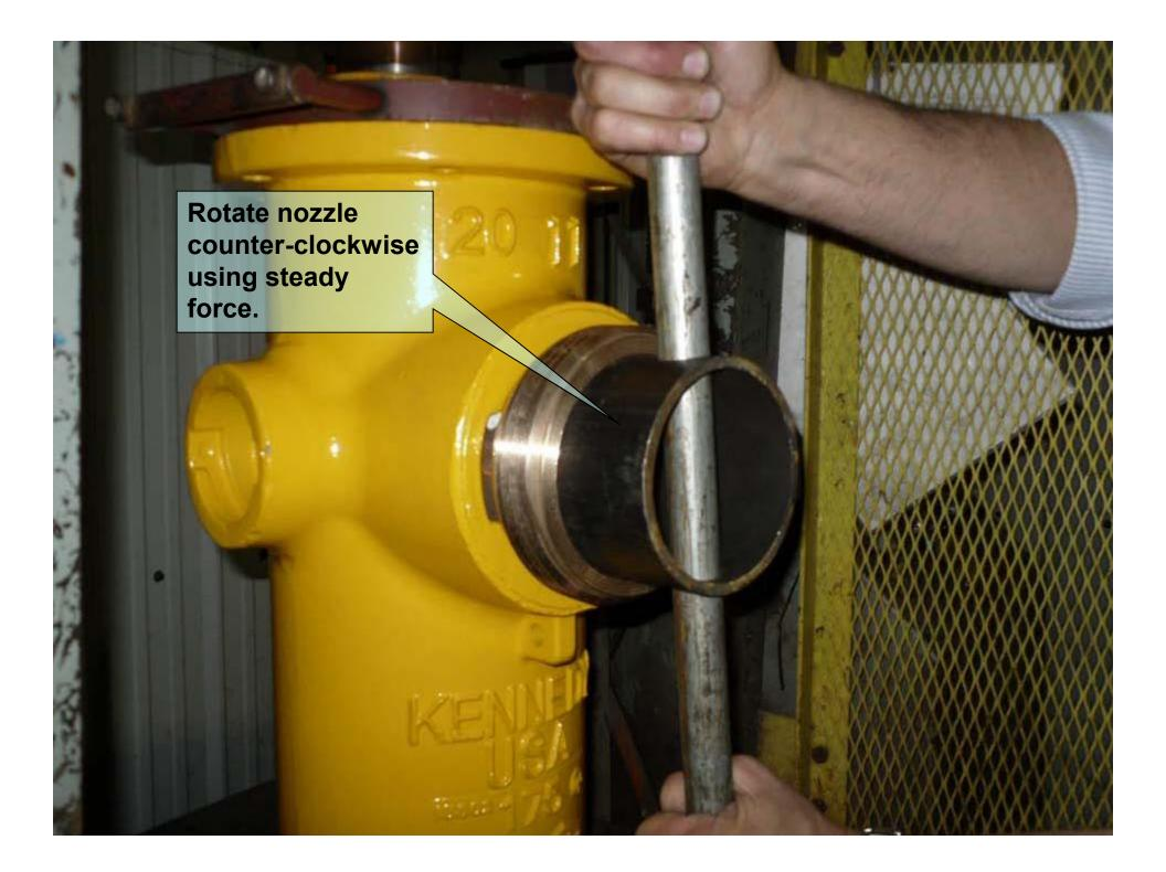
Notice as the nozzle is rotated, the end of set screw will begin showing while moving into its final position
